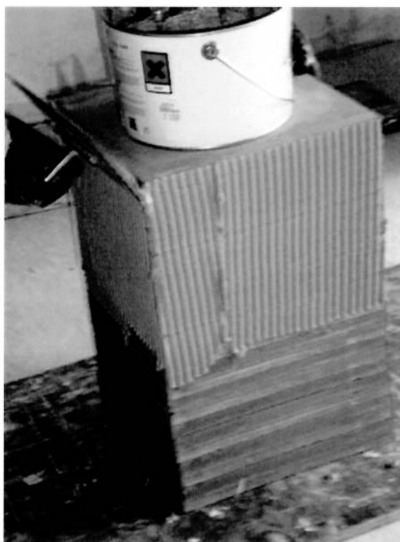
Figure 1 - Encollage des plaques
