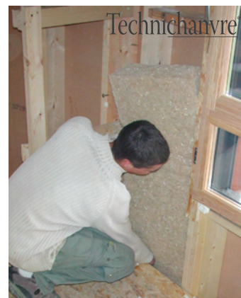
Pose TECHNICOOMPACT 100 en ossature
